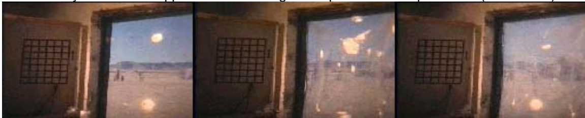
Laminated window exposed to blast pressures (condition 2).
